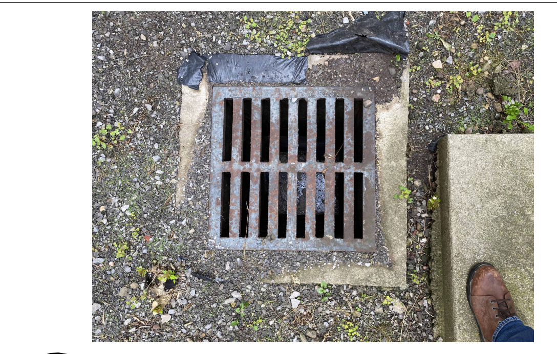
2 DEMOLITION PICTURE SCALE: NOT TO SCALE
