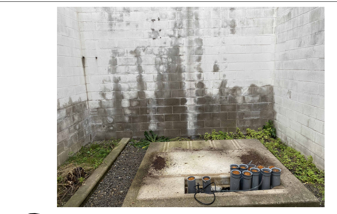
1 DEMOLITION PICTURE SCALE: NOT TO SCALE
