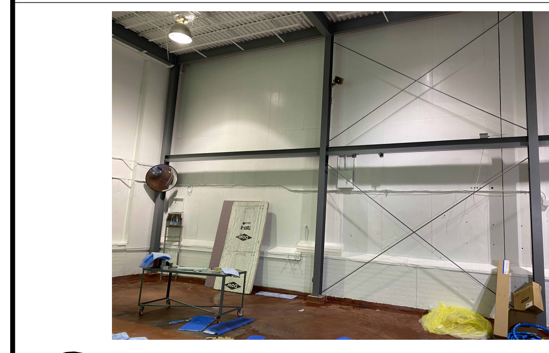
5 DEMOLITION PICTURE SCALE: NOT TO SCALE
