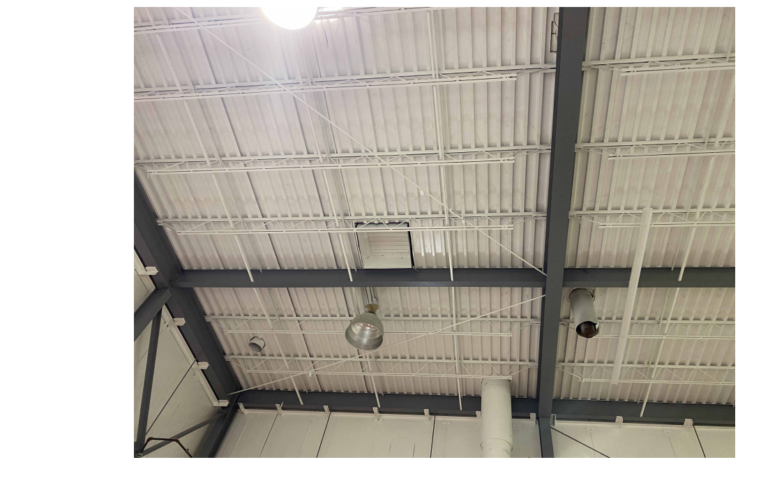
10 DEMOLITION PICTURE SCALE: NOT TO SCALE
