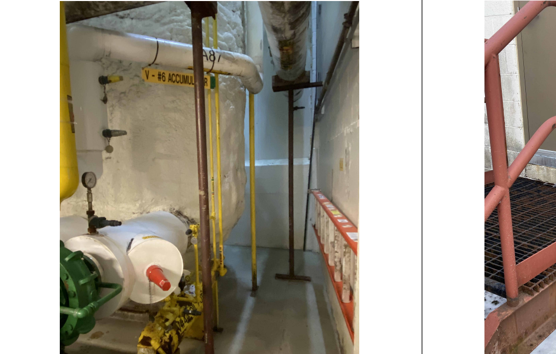
8 DEMOLITION PICTURE SCALE: NOT TO SCALE
