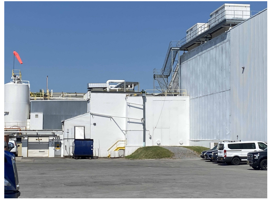
17 DEMOLITION PICTURE SCALE: NOT TO SCALE
