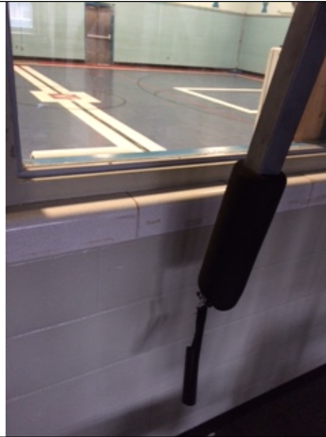
Room 33 – Glazed Block Window Sill
